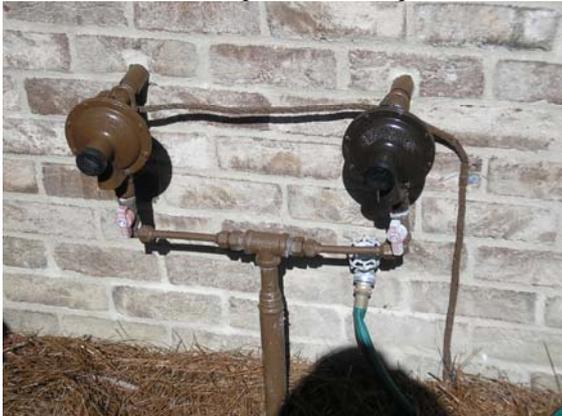
Figure 4. Bonding of incoming gas piping to LPS using main-sized conductor
