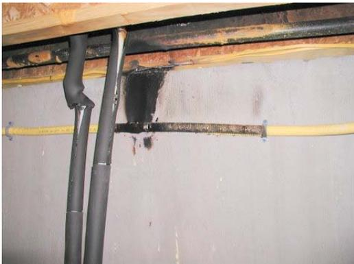
Figure 2. View of damaged CSST near two insulated vertical pipes below horizontal electrical cables and metallic water pipe
