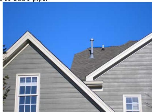
Figure 3. View of vent pipe on roof which served as the strike attachment point
