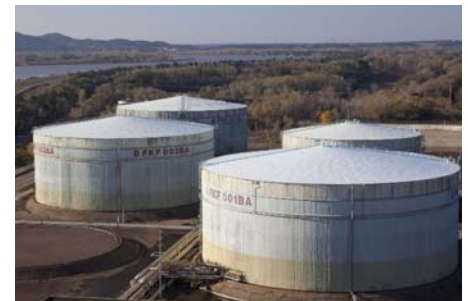
Fuel tanks – energie.edf.com
