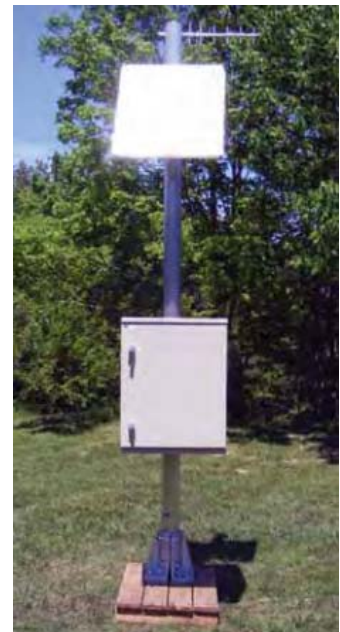
Dark Territory Wayside Installation PTC -in-a-Box
