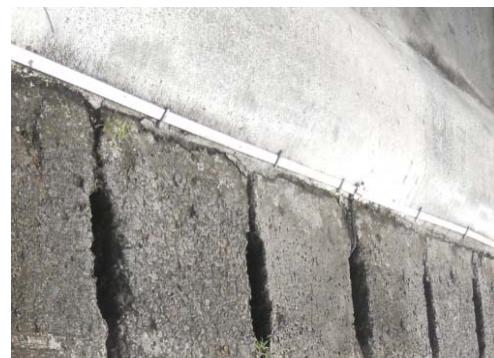
Copper conductor above cables routing, for cable protection
