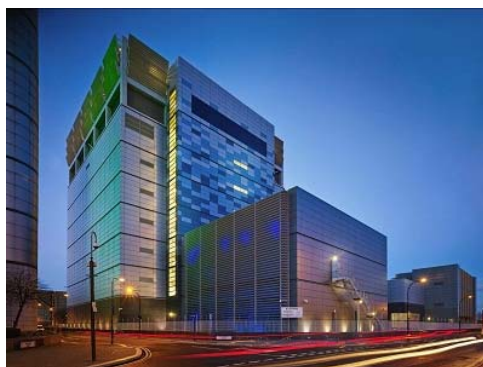
Data Center – Telehouse.fr
